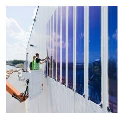
Equipped with a self-adhesive backing, the film can be applied directly to a variety of surfaces without further assembly efforts, and without affecting the structure underneath.
