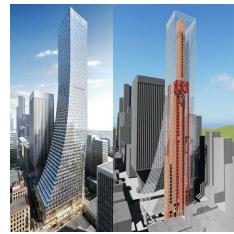
Californian digital manufacturing service provider 3Diligent has 3D printed 140 unique exterior curtain wall nodes for the Rainier Square Tower which is currently under construction in Seattle. Based on that requirement and the geometries of the nodes, 3Diligent created prototypes using investment casting and 3D printing. "We prototyped in both technologies and ultimately picked 3D Printing because of the dimensional accuracy and structural reliability it gave us.
